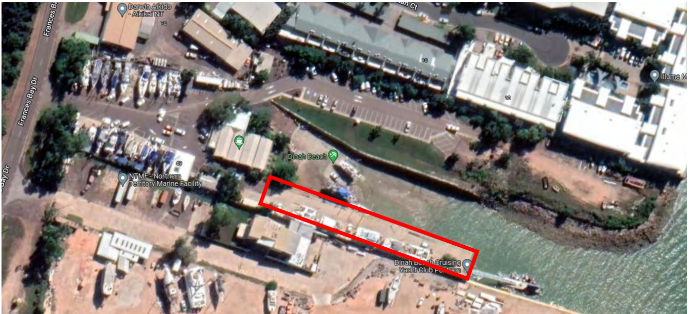
Figure 4 Concrete Wharf Location
